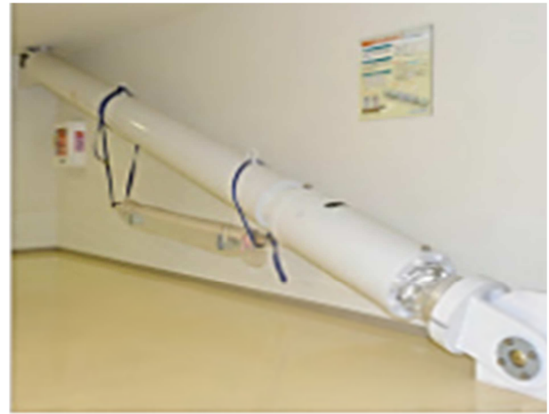
Figure 3. Installation of viscous damper to building [9, 11].
