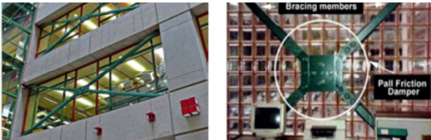
Figure 1. Installed friction damper to building [7].
