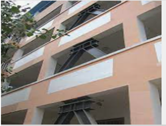
Figure 6. Metallic damper installed to the building [21].
