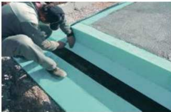
Figure 6. Placing of XPS isolation
