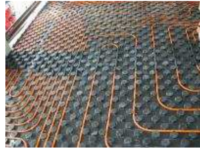
Figure 13. Underfloor heating system
