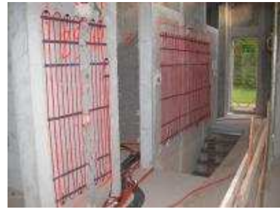
Figure 14. Wall heating system
