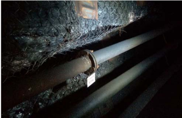
Figure 2. Large deformation occurred in the roadway.
