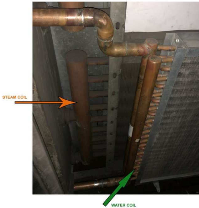
Figure 8. Steam and Hot Water Coils of the Unit Heater.
