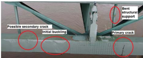
Figure 22. May 2019, I-40 Fatigue Crack – Earlier Bridge Inspection Video (Adapted from [37]).
