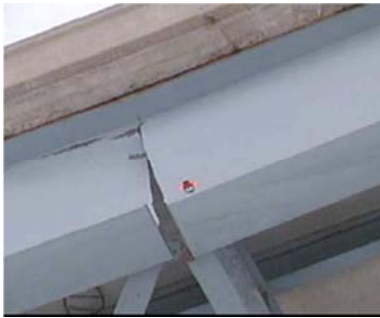
Figure 3. 2000, I-794 Hoan Bridge brittle fracture [15].
