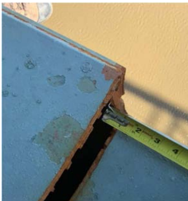
Figure 24. 2021, I-40 Fatigue Crack Dimensions [36].
