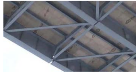
Figure 4. Hoan Bridge fracture propagated into two girders to cause brittle fractures [15].
