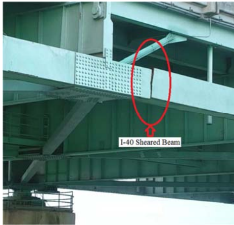
Figure 23. May 2021, I-40 Shear of Bridge Beam-Recent Bridge Inspection [36].
