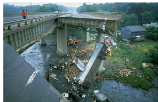
Figure 11. 1982 Mianus River Bridge collapse due to corrosion and fatigue [8].
