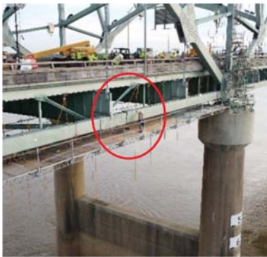
Figure 21. 2021, I-40 Fatigue Crack [36].
