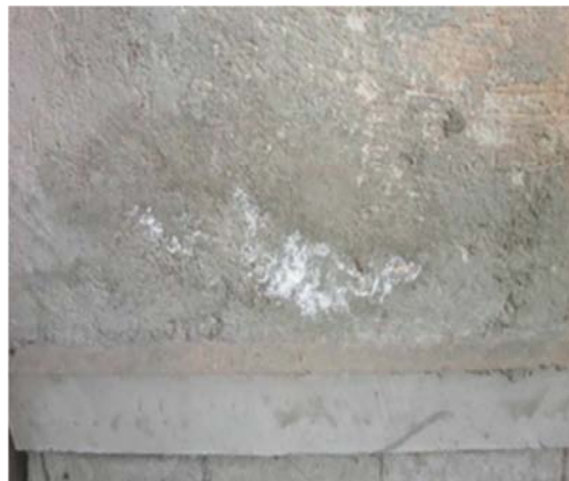
Figure 3. Efflorescence.
