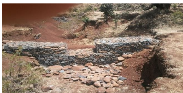
Figure 5. Checkdam constructed by the community at the study area for gully rehabilitation.
