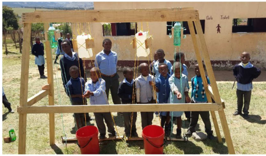
Figure 14. Press tap hand washing facility provided at the New Hebron School.
