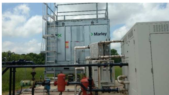
Figure 6. Cooling Tower.
