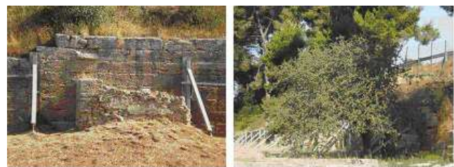
Figure 4. A anti-aesthetic retaining stabilization system with metallic pillars at the existing part of the ancient wall of Olympia.
