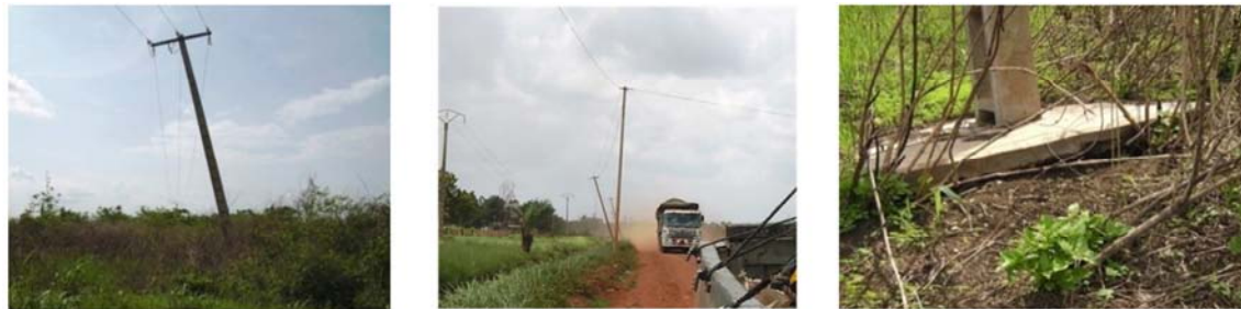
Figure 5. Tilt of electric poles and detachment of their sole in the region of Lama.
