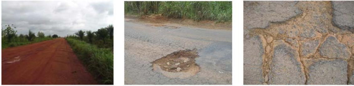
Figure 4. Degradation observed on pavements in the region of the Lama.
