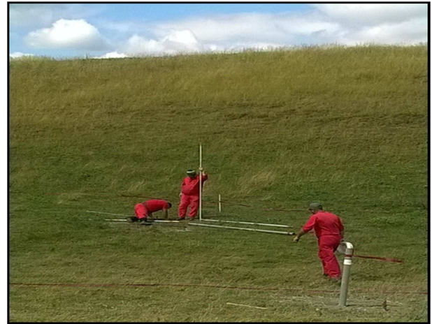
Figure 4. Loading the detonation holes at one of the sites.
