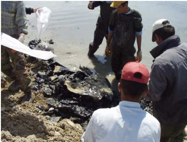
Figure 38. Recovering hardened oil on the shoreline, [11] and [12].
