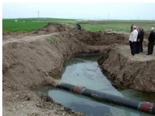
Figure 7. Repaired pipeline, [11] and [12].
