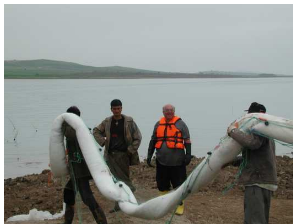
Figure 20. The fishnetted boom to the water for oil collection, [11] and [12].
