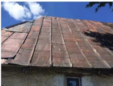
Figure 14. Retrofitted tin and existing shingle cover: effective protection against extreme weathering.
