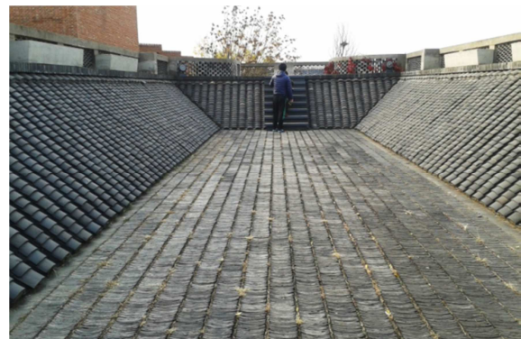
Figure 14. The newly-built V-shape roof.
