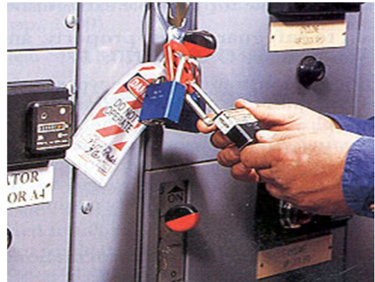
Figure 10. lock out/ tag out of electric panels.
