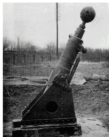
Figure 3. George Constantinescu's sonic tunnel: using just a trivial pistol cartridge, he was able to throw a 100-kilogram projectile at a distance of 1500 meters, perfectly silent, flame-free, smoke-free! In the contemporary era, the RAW system was proposed by the American company Brunswick Corporation. RAW is a self-propelled ammunition using a small solid-fuel rocket engine, while the device invented and made by George Constantinescu was thrown off by the rapid movement of a piston, which was in turn driven by the expansion of a high-pressure gas. In the case of the RAW system, the 140 mm diameter spherical projectile has a combat load (explosives, etc.) weighing 1.26 kg and a total weight of less than 4.5 kg with a maximum range of 2000 meters, of which the first 300-meter trajectory is straight, so shooting up to 300 meters does not require any shooting corrections. Ammunition total mass 4.27 kg, mass of projectile 3.82 kg, weight of combat load 1.26 kg. RAW Shooting System just looks like the sonic guns invented at the beginning of the second XX century by G. Constantinescu. Constantinescu's sonic gun (in both images) was able to completely silently throw a 100 Kg projectile at a distance of 1500 meters, but the performance limits of this type of weapon were (and are) far higher than what Constantinescu experienced in 1915. Source: Nic. P. Constantinescu, Encyclopedia of Technical Inventions , Royal Carol II Publishing House, 1939, and RAIDS Magazine , no. 82 of March 1993.
