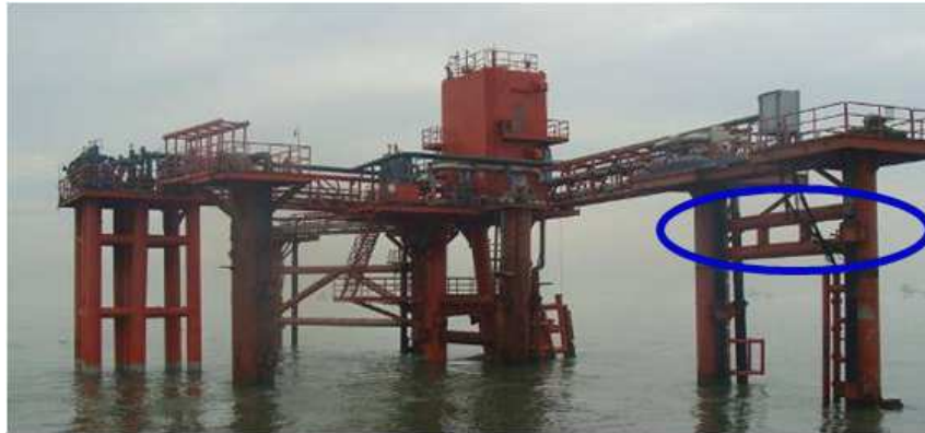
Figure 7. Tubular frame in offshore platforms.
