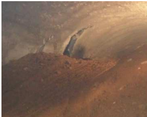
(d). The initial supporting cracking.
