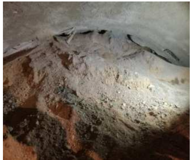
(a). Arch collapsed.
