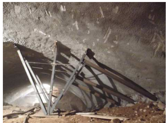
Figure 9. Temporary support in the hole.
