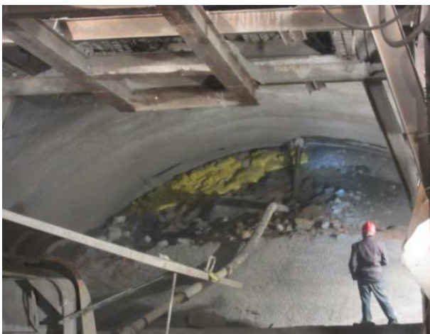
Figure 7. Sandbag plugging and backfill of the grouting.
