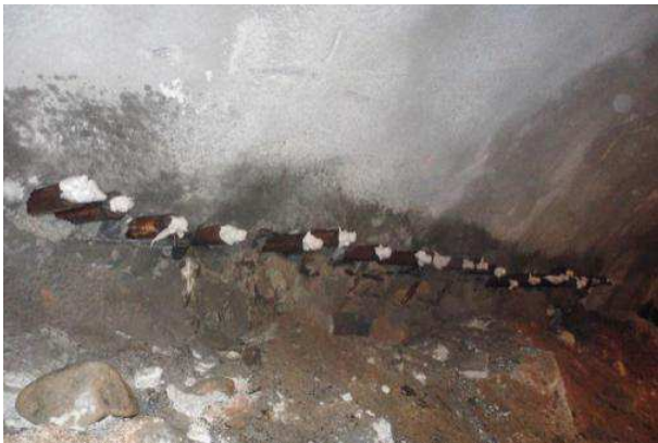
Figure 6. Lock foot anchor pipe.
