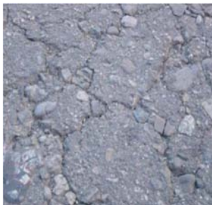
(1) Pavement spalling
