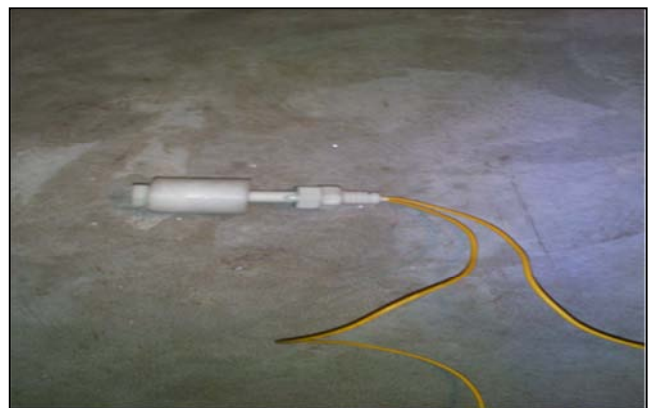
Figure 15. Floating Switch.
