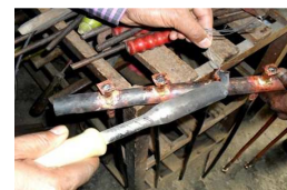
Figure 14. Soldering.
