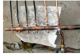
Figure 11. Attaching Copper pipes to the header pipe.
